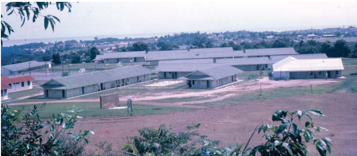
11 Indep Field Sqn lines looking out to the straits of Malacca. 2 Troop barracks in the foreground and NAAFI on the right. Beyond the tennis courts is the ORs mess.
