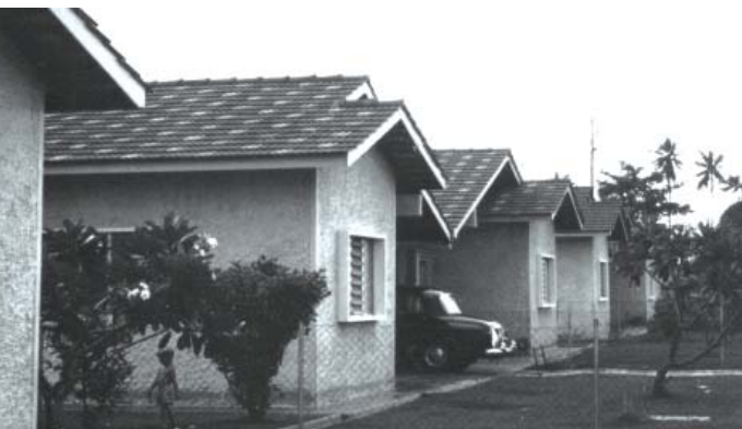
Typical married quarters in the purpose-built villages outside the garrison boundaries.
